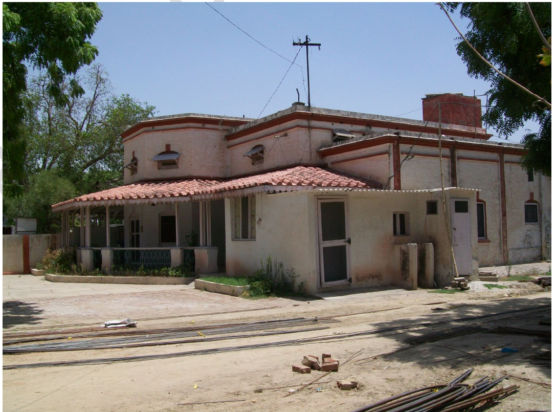
Figure 28: Residence of XEN Irrigation, Bathinda
